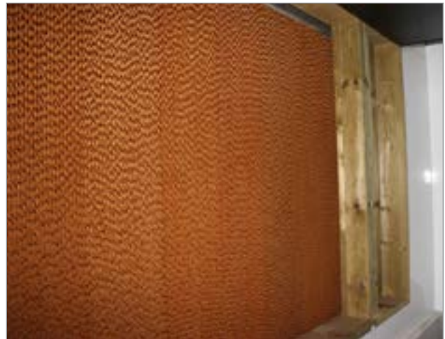
Figure 9. Inside surface of the evaporative cooling pad with the insulated door open.
