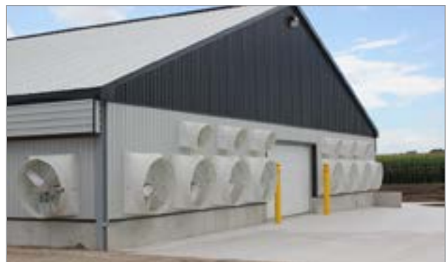
Figure 2. Exhaust fans across the end wall of the barn.
