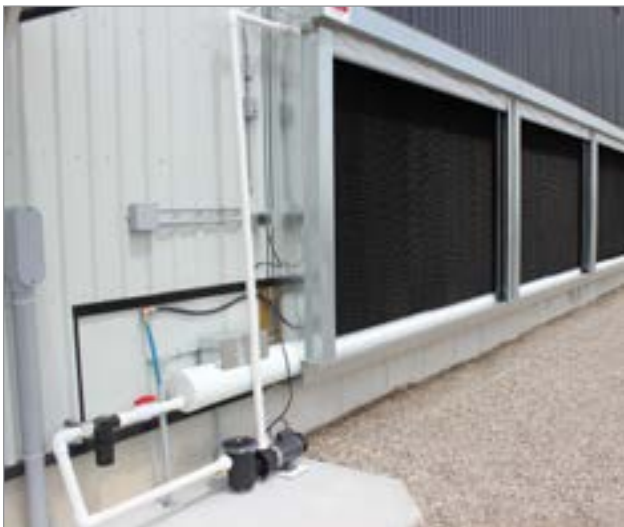
Figure 7. Evaporative cooling pad, showing circulating pump, cooling pad, fresh water feed pipe (blue pipe) and filter.
